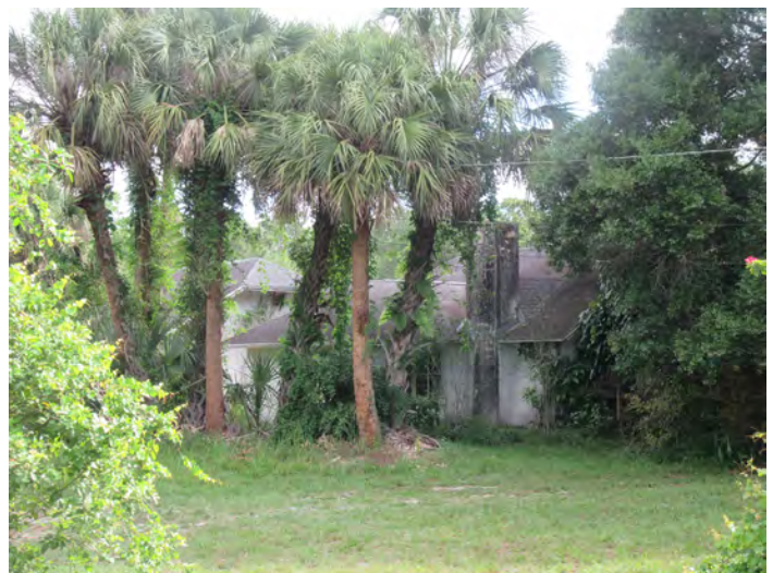
8BR04378_f Facing Northeast
