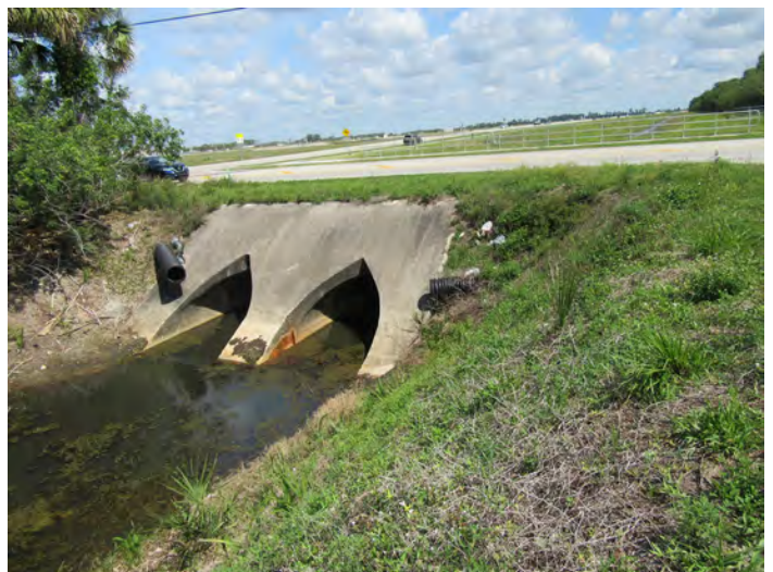
8BR04374_f Facing Northwest
