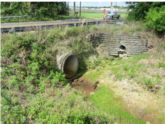
8BR04379_e Facing Southwest
