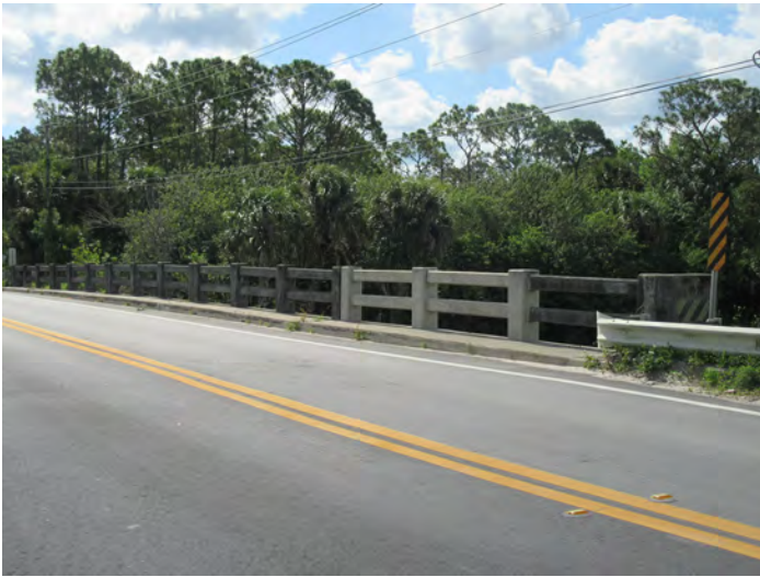
8BR04380_g Facing Southeast
