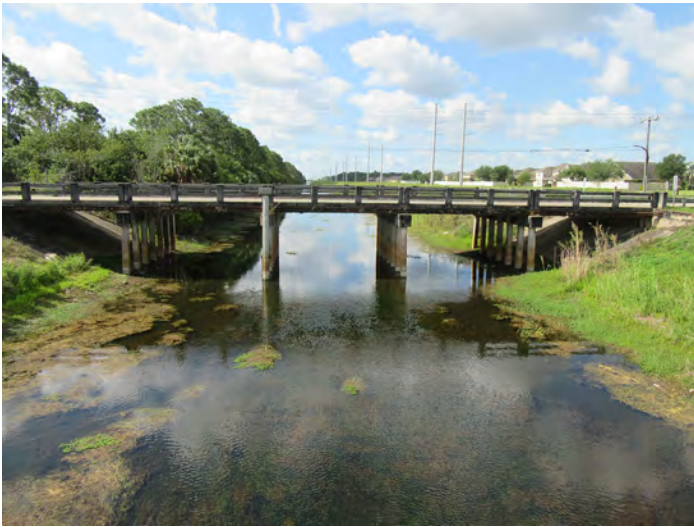
8BR04380_a Facing South
