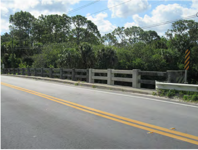
8BR04380_g Facing Southeast
