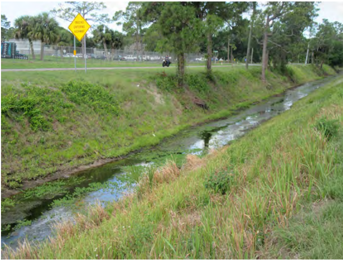
8BR03535_a Facing Southwest
