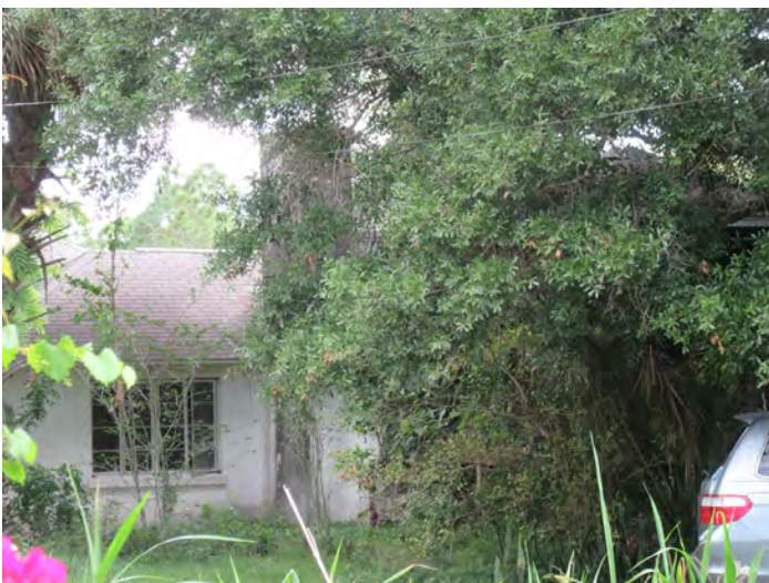
8BR04378_e Facing North
