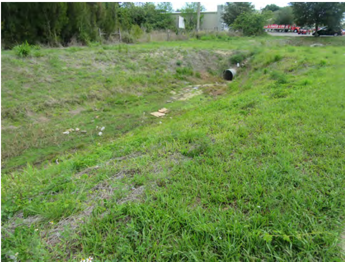
8BR03535_i Facing Northeast
